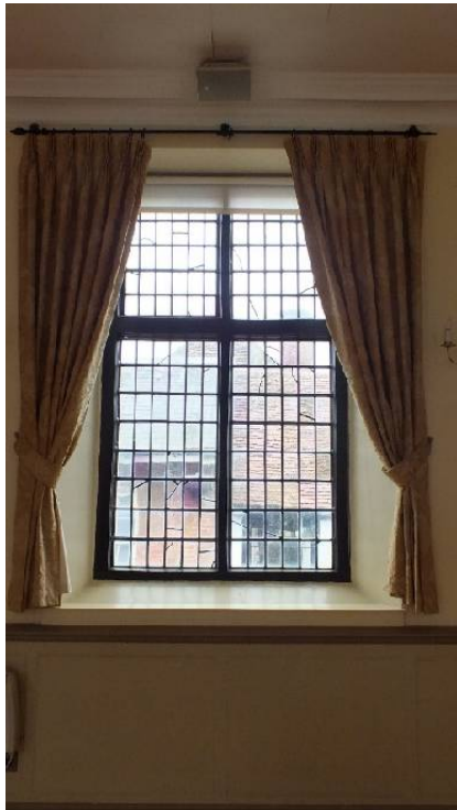
Figure 27 Example of the windows in the hall with their lead cams and small glass panes.
