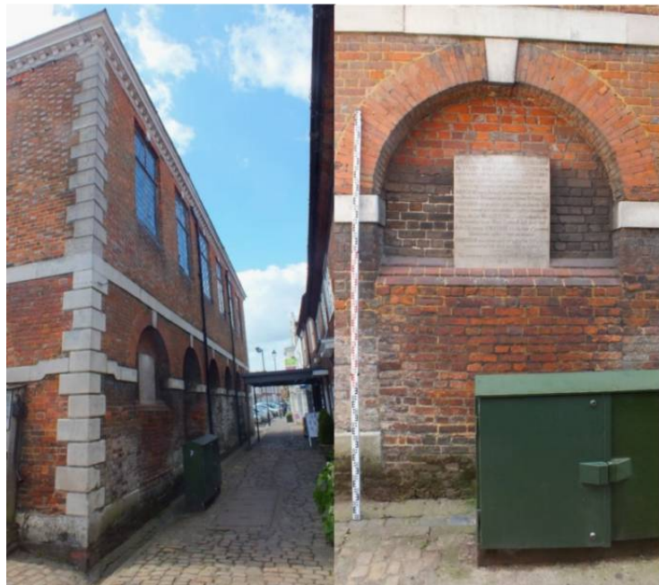
Figure 15 (a) Left Hand Side: Showing Northern Elevation of Market Hall with bricked in first arch and drainpipes. It also highlights the difficulties with photography relating to this building. (b) Right Hand Side: Showing detail of first arch and the shelf like pattern of the bricking up and the Amersham Society Plaque that commemorates the Domesday entry of Amersham town.
