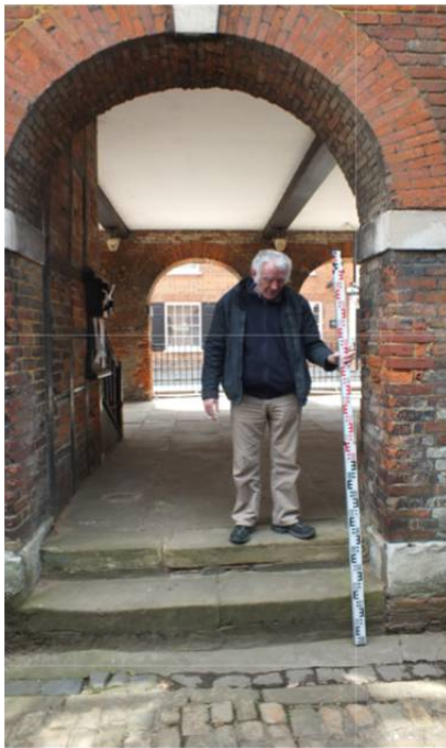
Figure 14 Stone Steps on Northern Elevation of building
