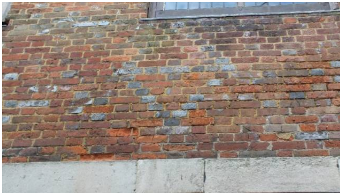
Figure 17 Diamond Pattern of header burnt bricks on North elevation
