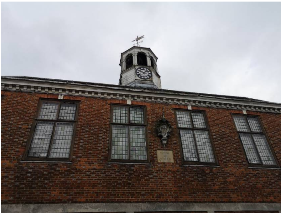
Figure 4 Photograph of Southern elevation showing upper floor windows.
